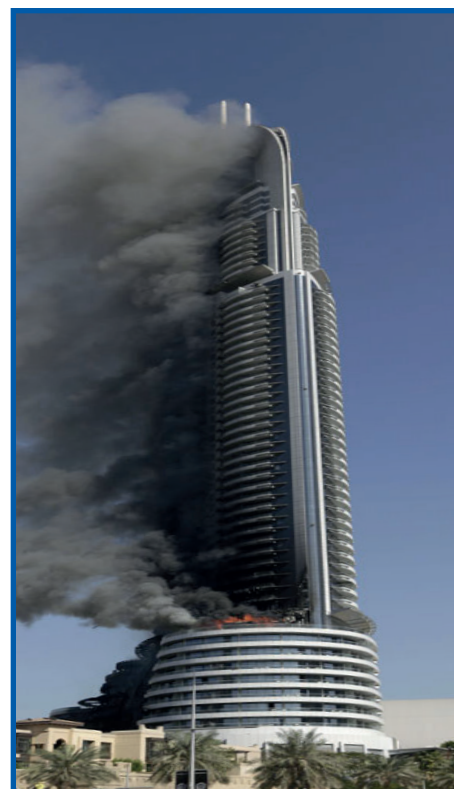
On December 31st 2015 at 9:30 pm a major fire broke out in the Address Downtown hotel in Dubai, causing one death and 60 injuries
