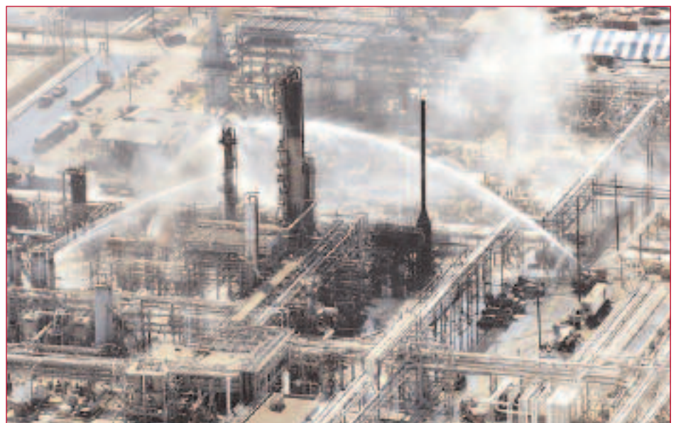
Aftermath of the Texas City refinery explosion, 23rd March 2005
