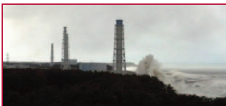
The Japanese tsunami strikes the turbine building of the Fukushima Daiichi nuclear power plant
