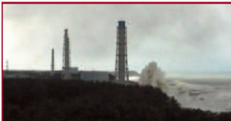
The Japanese tsunami strikes the turbine building of the Fukushima Daiichi nuclear power plant
