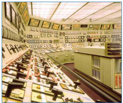
The design philosophy of any alarm system is to alert the operator to a plant condition that has reached or exceeded a pre-defined limit, so that he or she can take action or monitor any automatic response.
